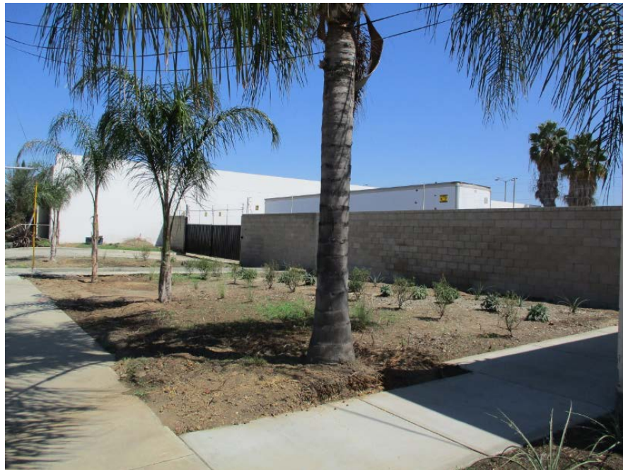
Figure 5: Fencing removed, 8' block wall constructed, landscaping installed
