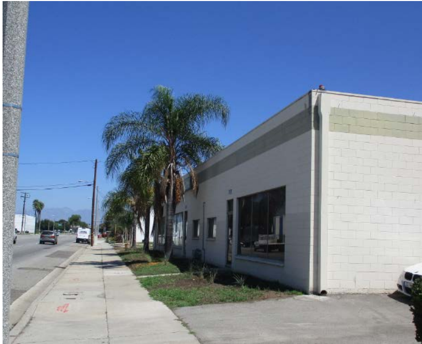
Figure 7: Pole sign removed, landscaping installed
